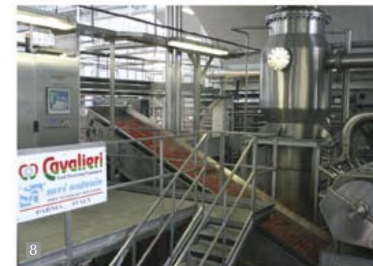
Photo 8 Control Panel with PLC and System Management with Industrial PC
